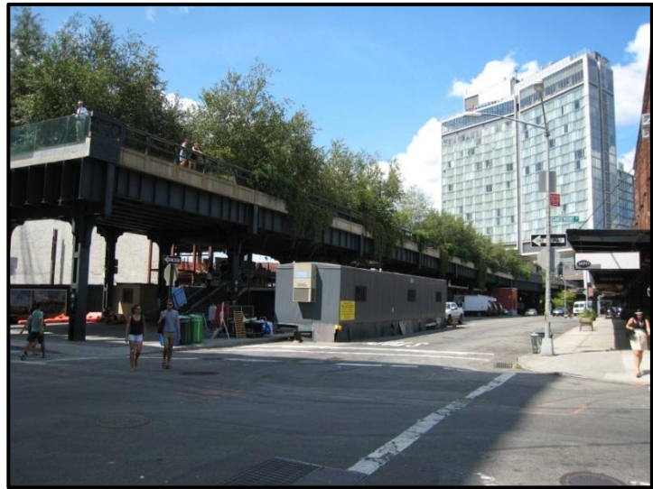
Figure 10: View of the highline walkway taken from across street from the southeast corner of the site. Photo taken by Vincent Rossi.
